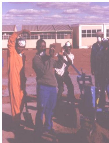
Figure 4 Training of a group in the production of cement stabilised compressed earth blocks (CEB) in Bankhara Bodulong.
