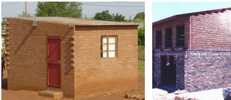
Figure 5 Use of CEB bought from local entrepreneurs for a self-help house and the local school in Bankhara Bodulong
