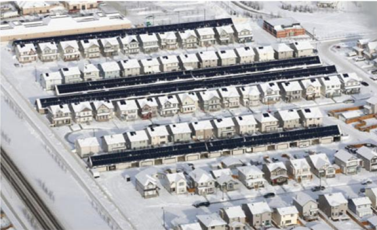
Figure 6 Solar district heating with annual heat storage. Drakes Landing, Canada (photo: AEE-Intec)
