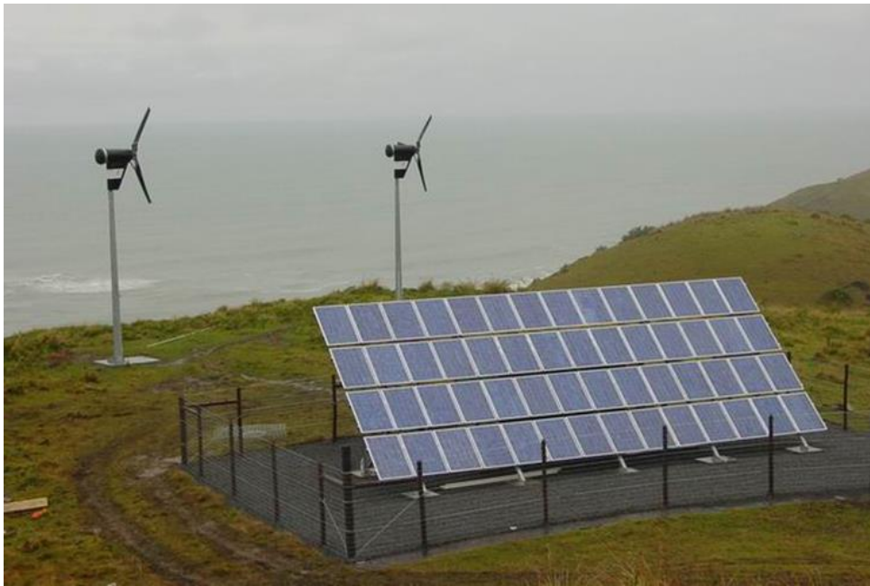
Figure 2 Hybrid mini-grid system at Hluleka Nature Reserve
