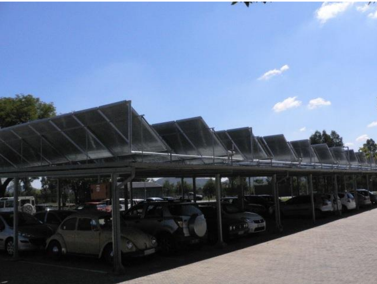
Figure 7 The 700m 2 SWH system at Onderstepoort, University of Pretoria doubles up as protected parking (photo: HolmsandFriends)
