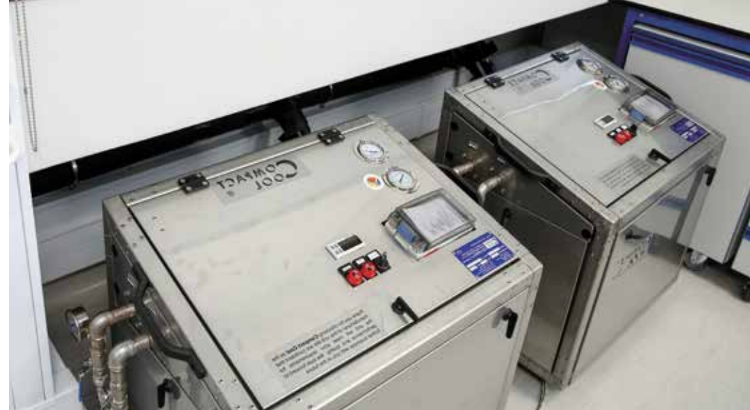
Equipment used to extract heat from laser sources.
