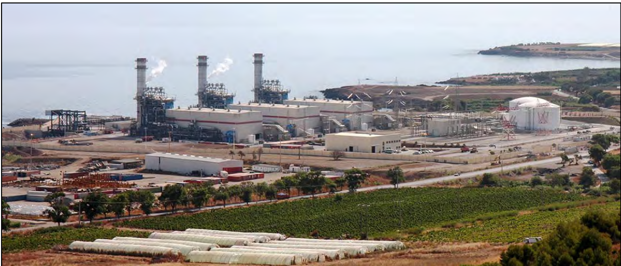
Figure 2.12: Existing CCGTs at Wilaya of Tipaza, Algeria (3x400 MW configuration, 1 227 MW Shariket Kahraba Hadjret En Nous power station) (Mubadala Development Company PJSC, 2016). Similar plants will be part of new CCGT capacity planned for in the IRP 2010.
