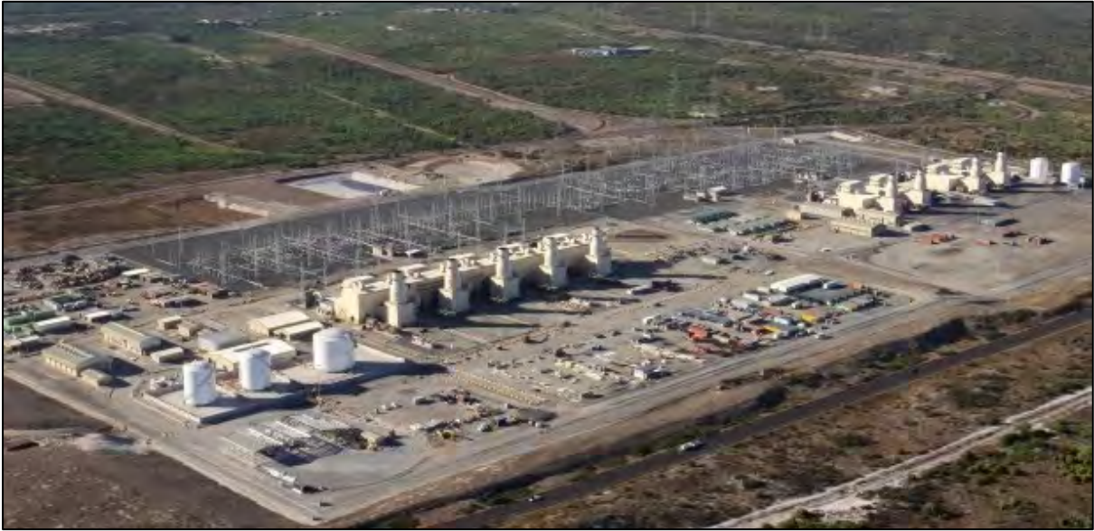
Figure 2.11: Existing OCGTs at Atlantis, South Africa (9 x 148 MW, 1 327 MW Ankerlig power station) currently running on diesel (Eskom Holdings SOC Ltd, n.d.). Similar plants will be part of new OCGT capacity planned for in the IRP 2010 but will run on natural gas.
