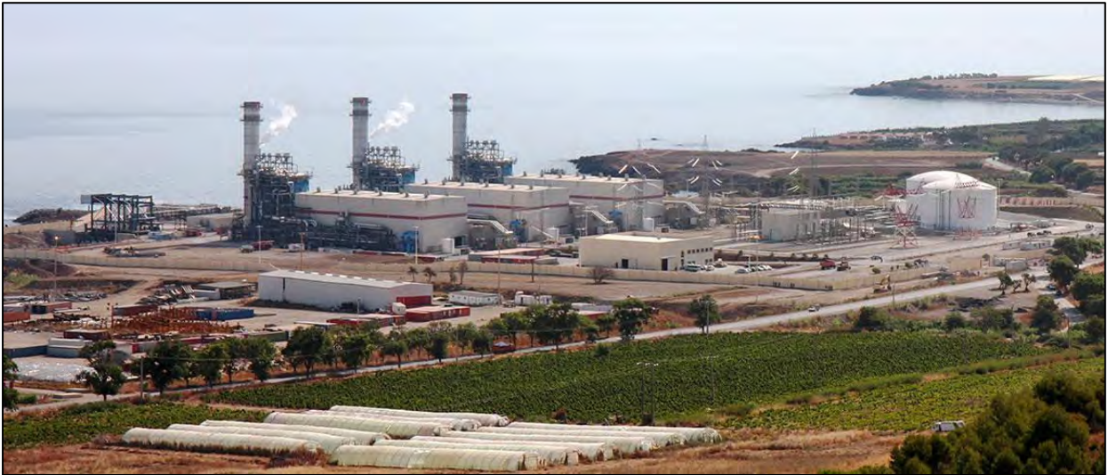
Figure SPM 2.1: Power plant with three combined cycle gas turbines (CCGT) located in Algeria. Similar plants are planned as part of new CCGT capacity under the IRP 2010, regardless of whether exploitable shale gas is found in South Africa or not (Mubadala Development Company PJSC, 2016).
