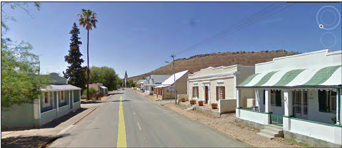
Figure 15.6: The well-preserved streetscape of Church Street, Victoria West.
