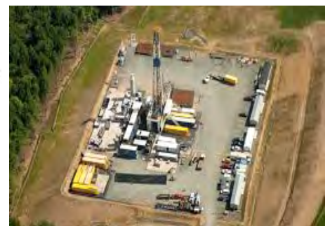
Figure 14.7: Typical wellpad with drilling rig (rsfb.org.uk)
