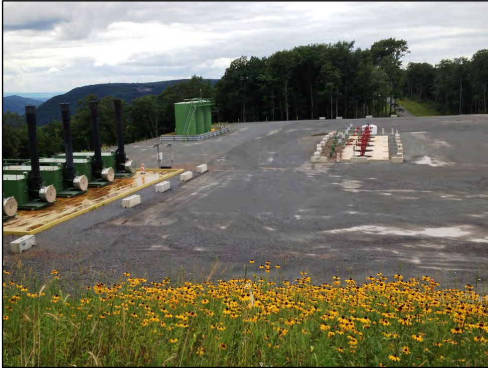
Figure 1.38: Example of a shale gas compressor station situated at a wellhead complex. Tanks used to store produced water and condensate, separated from ‘wet gas’, are shown located towards the top left of the photograph (Source: Tom Murphy (n.d.), Pennsylvania State University, USA).
