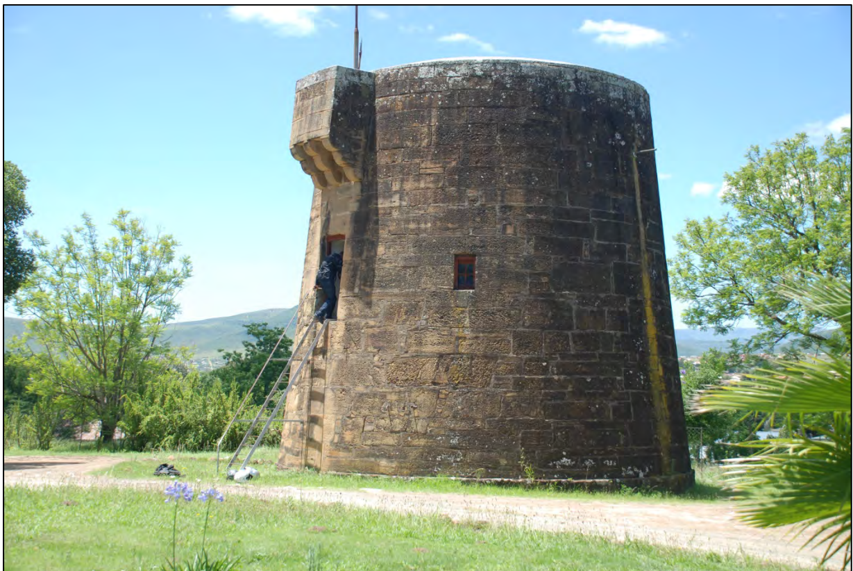
Figure 15.4: Martello Tower, Fort Beaufort.
