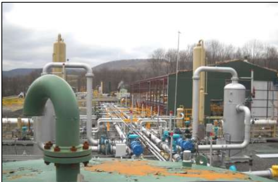
Figure 1.39: Example of a centralised gas compressor station. Compressed gas would be exported from this facility, via pipeline, to a downstream facility such as a CCGT power station (Source: Tom Murphy (n.d.), Pennsylvania State University, USA).
