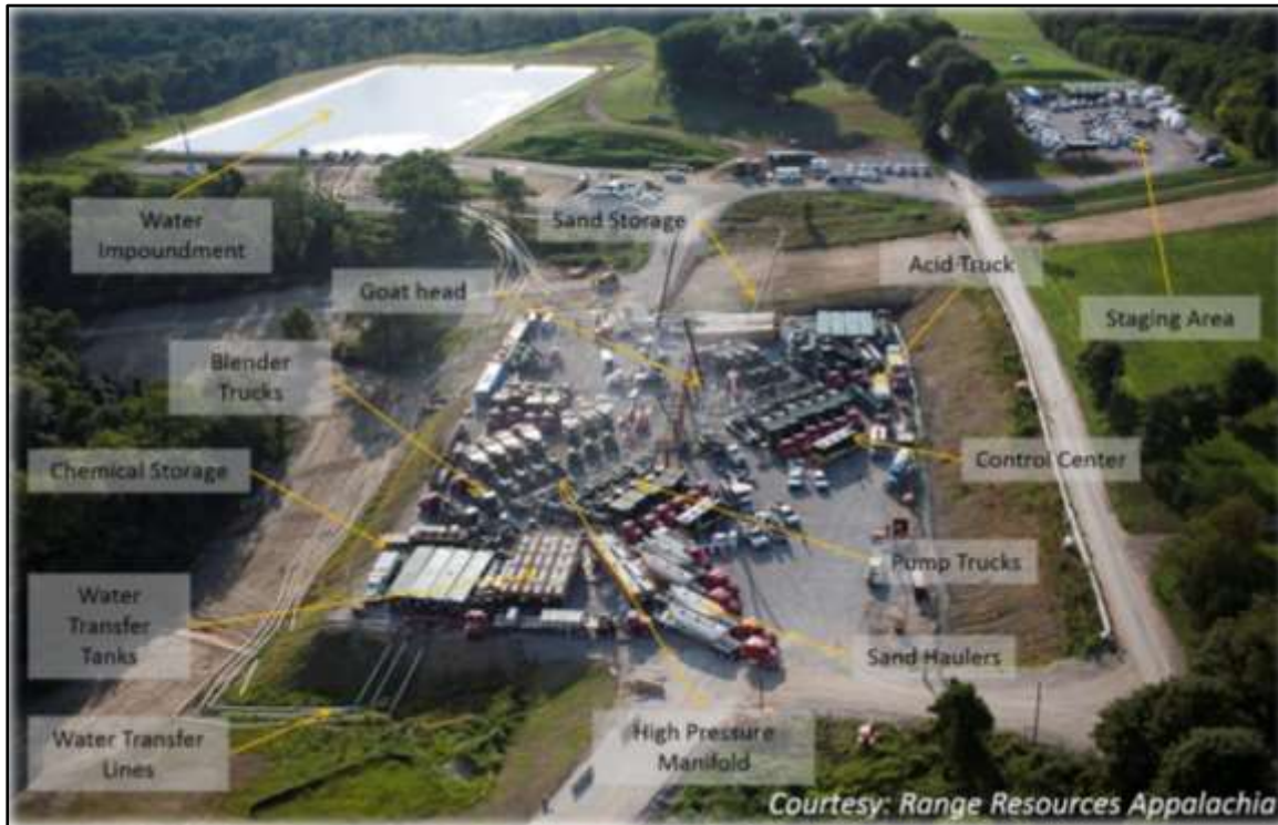
Figure 1.29: Example of a fracking process underway in Appalachia, with the main equipment and facilities involved indicated (Source: Range Resources Corporation).
