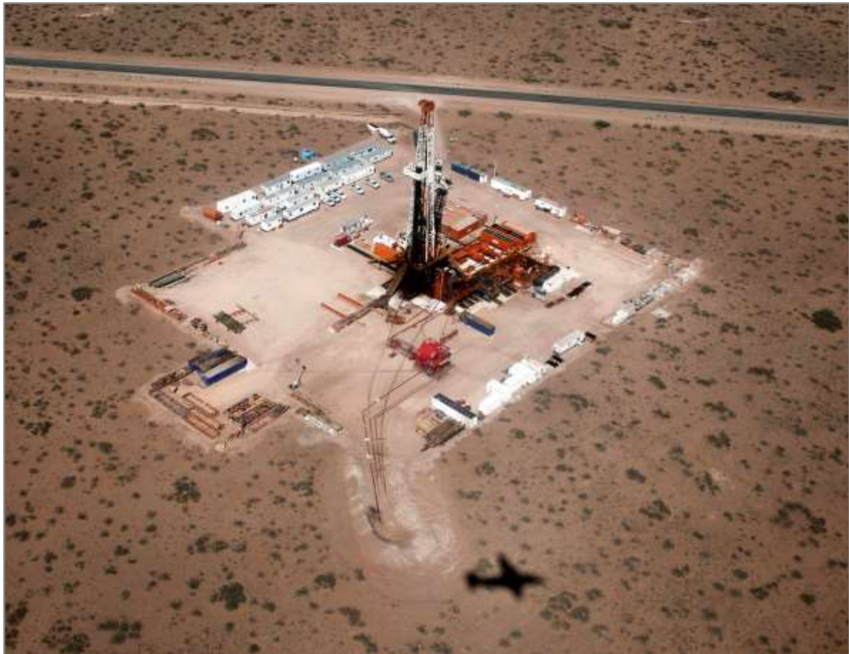
Figure 1.23: A typical wellpad layout with drilling and supporting infrastructure in place within an arid environment in Argentina, similar to what may be encountered in the Central Karoo ( Source: REUTERS, http://www.vcpost.com/articles/5923/20120925/sidewinder-drilling-to-buy-union-drilling-for-139-mln.htm ).
