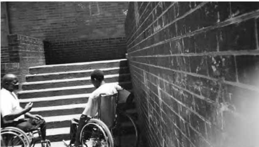
Figure 23.8: Saulsville railway station: no access
