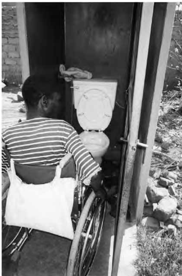
Figure 23.2: Inaccessible toilets in RDP houses
