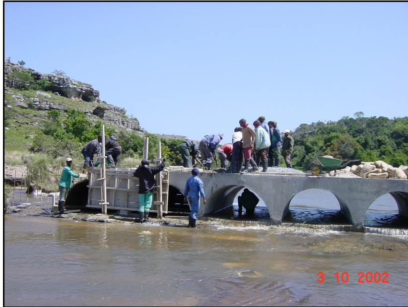
Figure 2. Construction of Causeway by Local Semi-skilled Labourers
