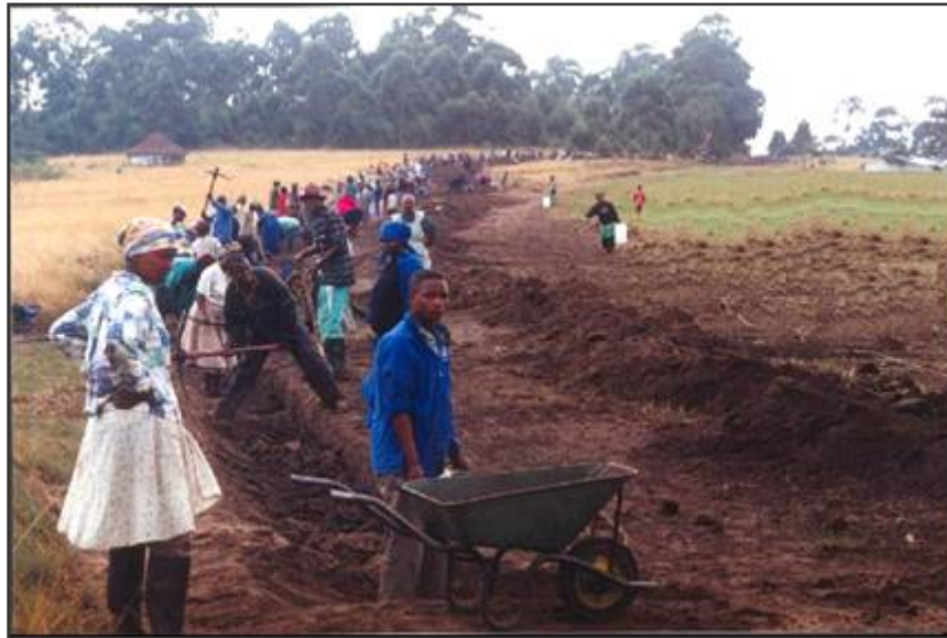
Figure 1. Labour Force Constructing the Road Formation
