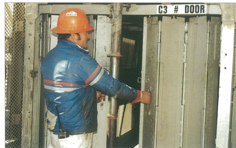
Uniquely designed mine hoist cage door
