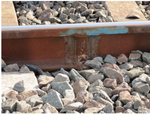
Figure 8 Thermite weld and measured reflection at 300m.
