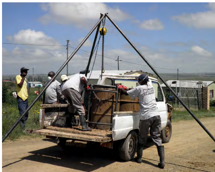
Drums, filled with sanitation waste from households in Dutywa, are loaded for safe disposal.
