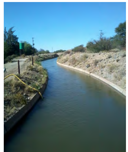
Below: A typical irrigation water canal.
