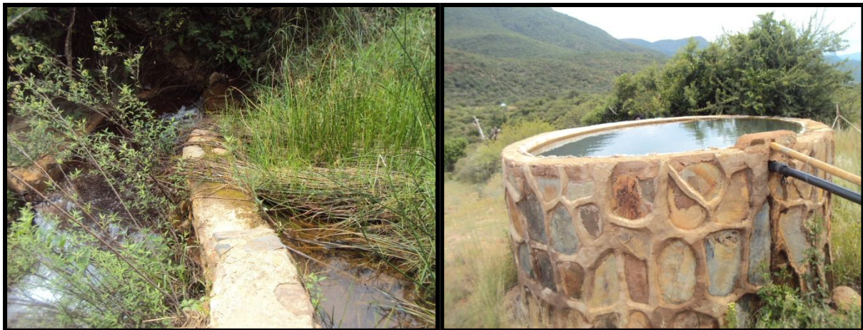
Figure 1: The mountain water scheme weir (left) and reservoir (right)
