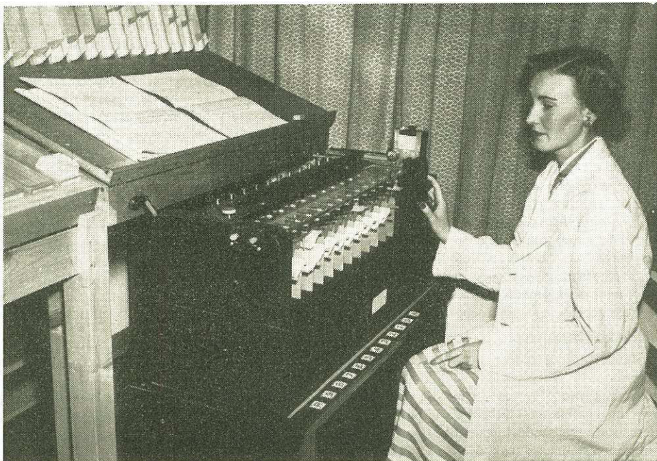
A machine for the sorting of punched cards containing psychological test data.
