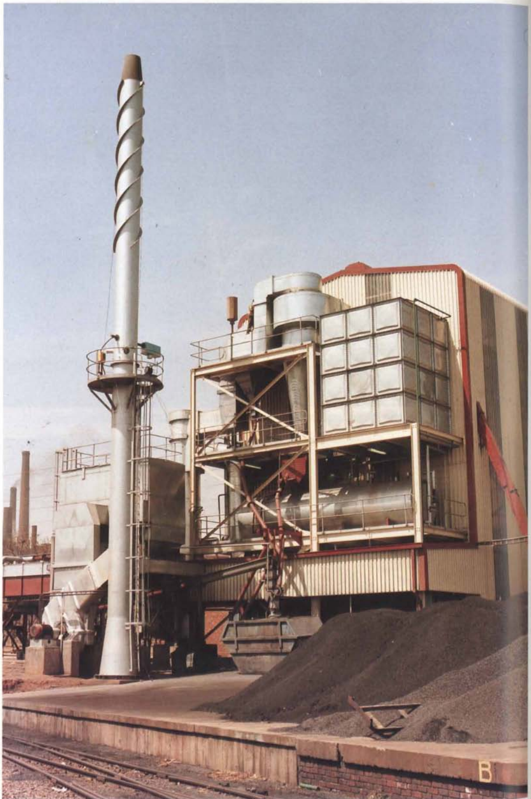
Fluidised bed combustion technology was developed for the burning of duff and discard coal, coal slurries, organic sludges and biomass waste. An associated hot gas generator and a boiler developed for different companies both received awards from South African professional engineering institutes.
