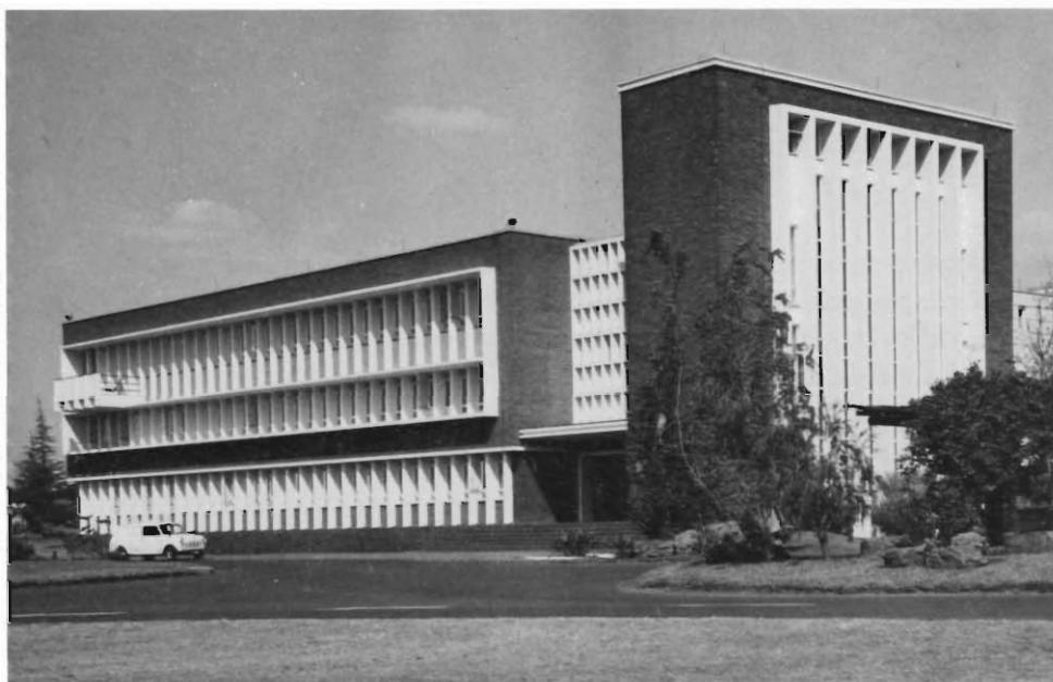
The Administrative Services Department building
