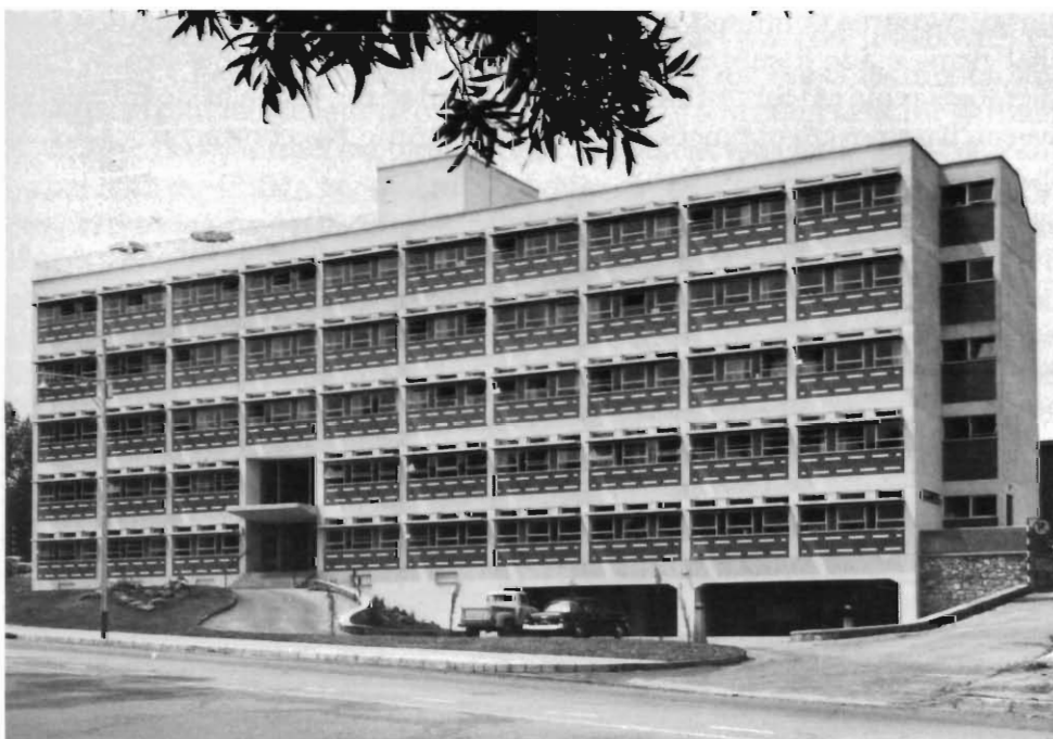
The headquarters of the National Institute for Personnel Research in Empire Road, Johannesburg, since 1962.
