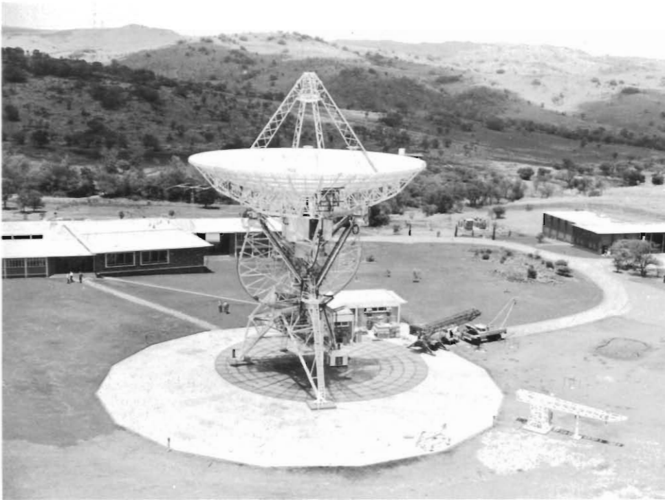
Deep space probes were accessed and tracked by means of this 26-m dish antenna at Hartbeesthoek near Krugersdorp.
