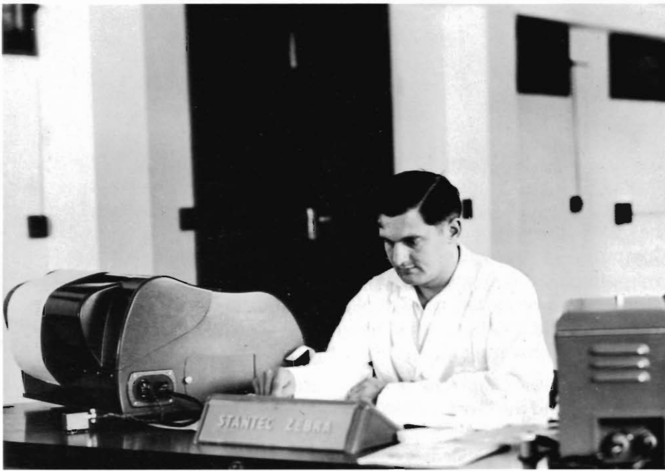
The first electronic digital computer, code-named ZEBRA, was installed at the CSIR in 1958 to facilitate automation in research. It recorded data on punched paper tape, which could then be fed into the computer.
