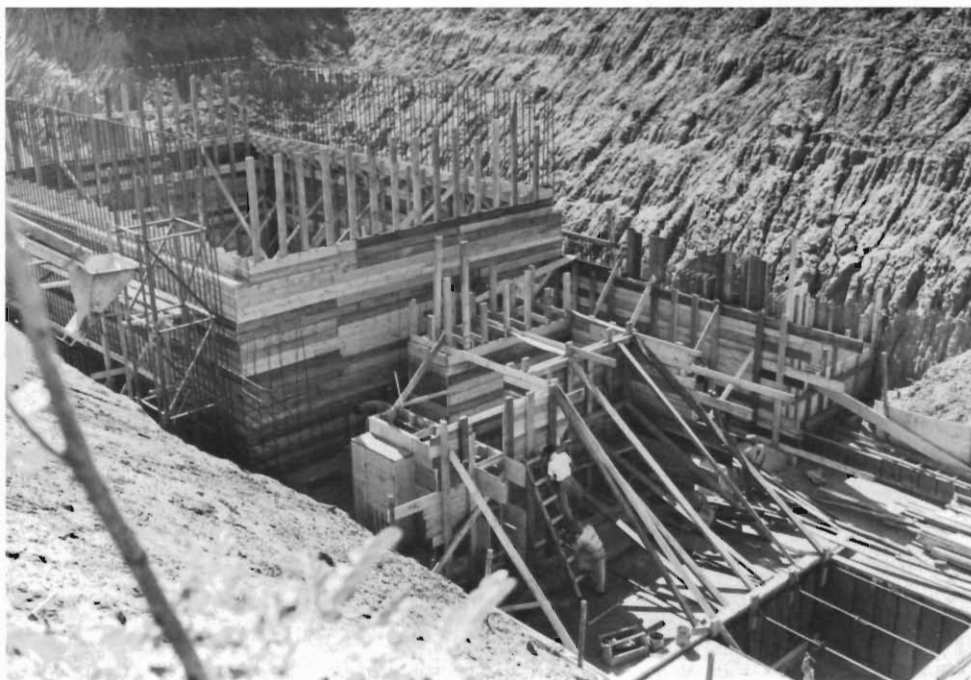
The underground cyclotron hall under construction at Scientia.
