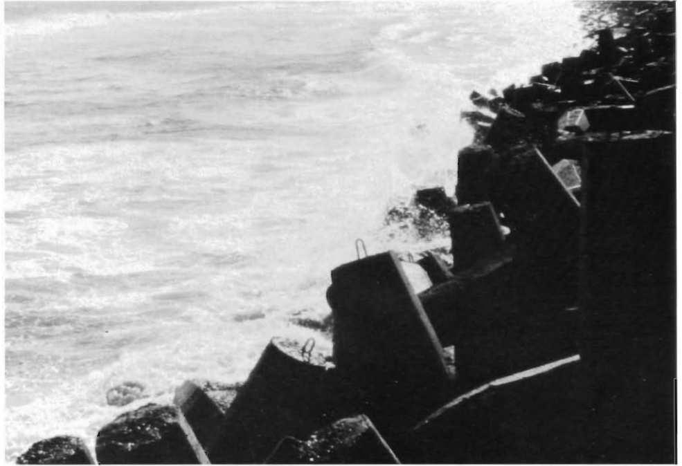
'Dolos' breakwater armour units.
