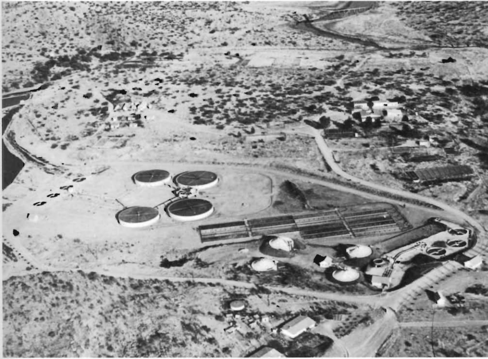
The water reclamation plant near Windhoek in South West Africa.
