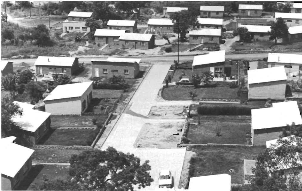
Part of the KaNyamazane demonstration project near Nelspruit, incorporating an innovative lay-out, alternative house-types designed and sited in such a way as to facilitate easy expansion and improvement.
