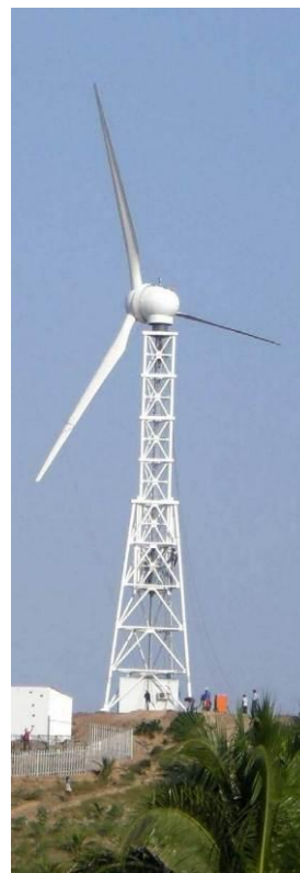
Figure 2: Adventure Power's 300kW wind turbine.
