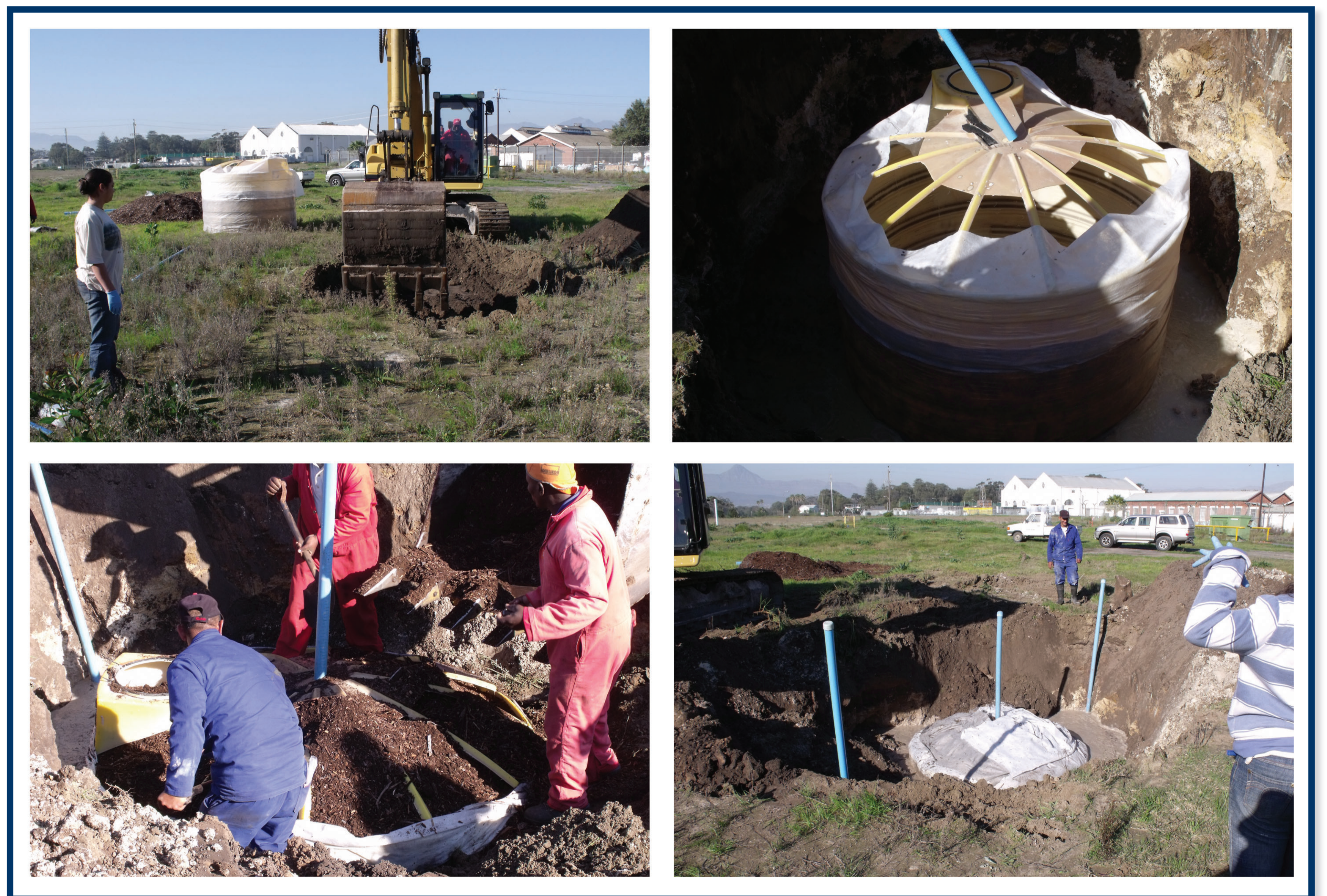
Figure 3: Steps during the emplacement of the vessel of carbon amendment for denitrification
