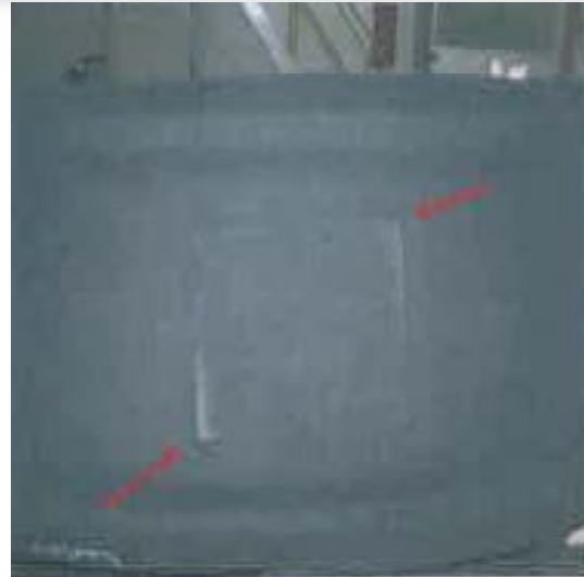
Impression mark visible after load testing
