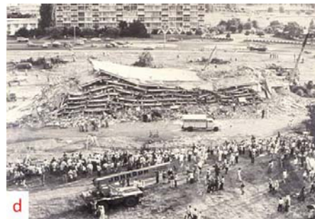
(d) Collapse of block of flats in Welkom following M_L = 5.2 tremor in 1976 (Durrheim, 2010).
