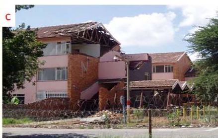
(c) Surface damage in Stilfontein after M_L=5.1 event in March 2005 (Durrheim, 2010).
