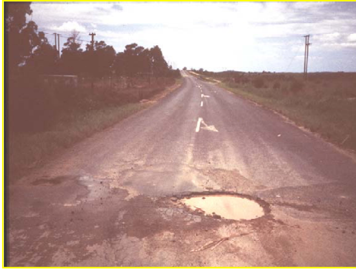
FIG. 7. Typical pothole with water in a thinly surfaced road.
