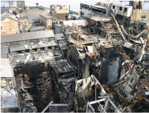
Figure 1—Aftermath of aluminium dust explosion at Hayes Lemmerz International-Huntington foundry 6
