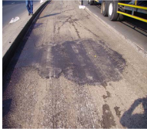
Figure 5: Milled out section levelled with a scratch coat for a smooth surface
