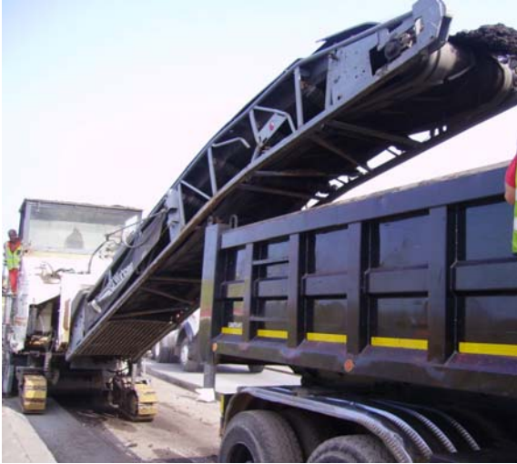
Figure 4: Milling of the existing asphalt layers
