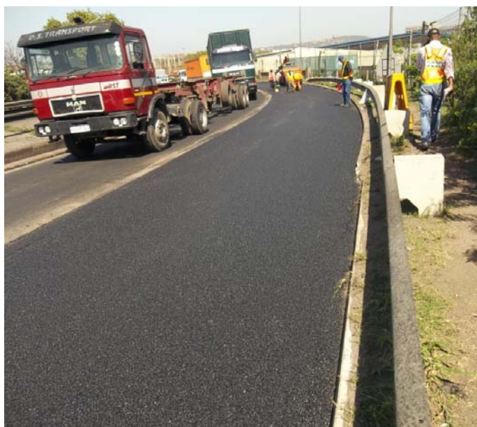
Figure 8: Finished surface of HiMA layers
