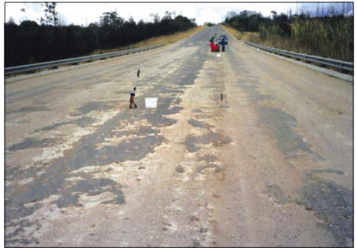
Photo 3 Loss of most of prime under light traffic on same road as in Photo 4
