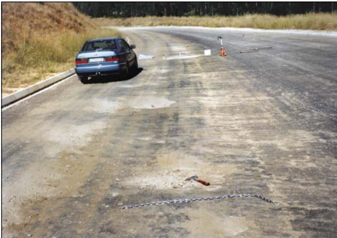
Photo 4 General view of weak, carbonated, primed 3% cement-stabilised weathered granite base disintegrating under light traffic and showing chain drag in foreground
