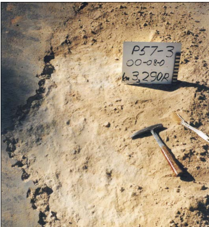
Photo 6 Close-up of Photo 5 showing exposed harder base after loose to weak upper 25 mm of carbonated base had been hand-broomed off
