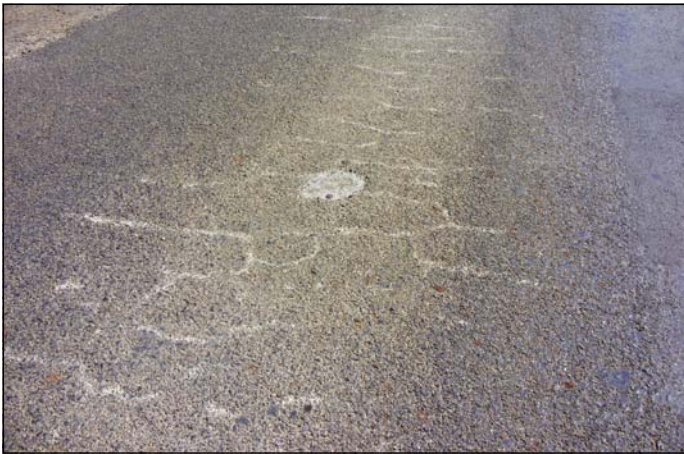
Photo 2 Fatigue cracking and pumping on a recently constructed main road – possible weak interlayer directly under the surfacing seal (courtesy of Dr P Paige-Green)
