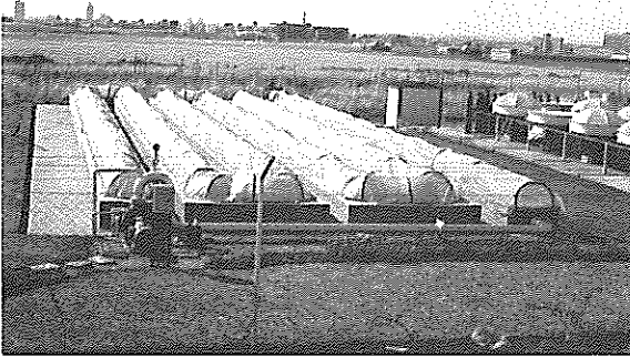
Fig. 6.1. "Closed" algal ponds at the University of the Orange Free State, Bloemfontein, South Africa. Left: 100 m 2 pond; right: some of the miniponds.
