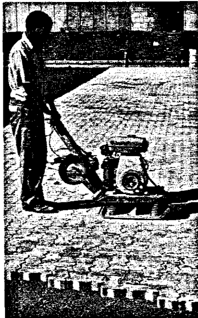
Figure 12 - The use of a light plate vibrator to compact the sand bed
