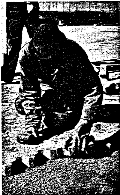
Figure 11 : Placing the units on the sand bed
