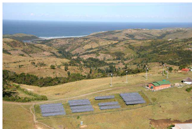
Figure 8: Lucingweni 86 kW hybrid mini-grid
