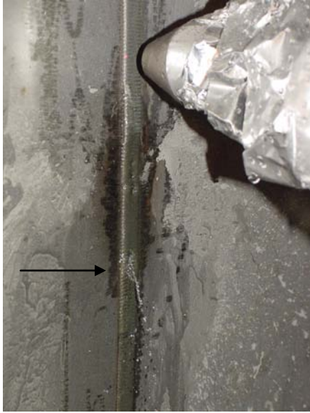
Figure 3: Crack sealing without peening prior to cladding.
