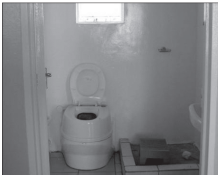
Figure 8: Urine diversion toilet and a shower in a Hull Street house Source: Matsebe, 2008
