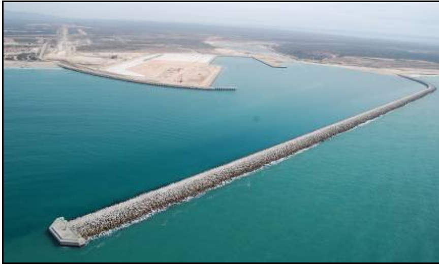
Figure 3: Dolos breakwaters at the Port of Ngqura
