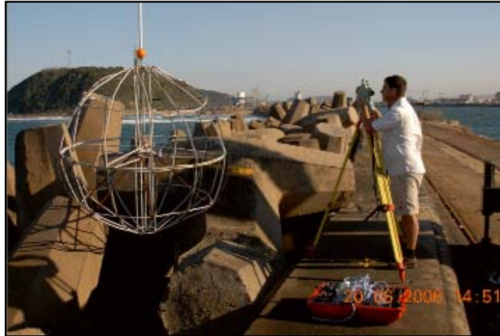
Figure 5: Crane and Ball Survey of Breakwater Profiles
