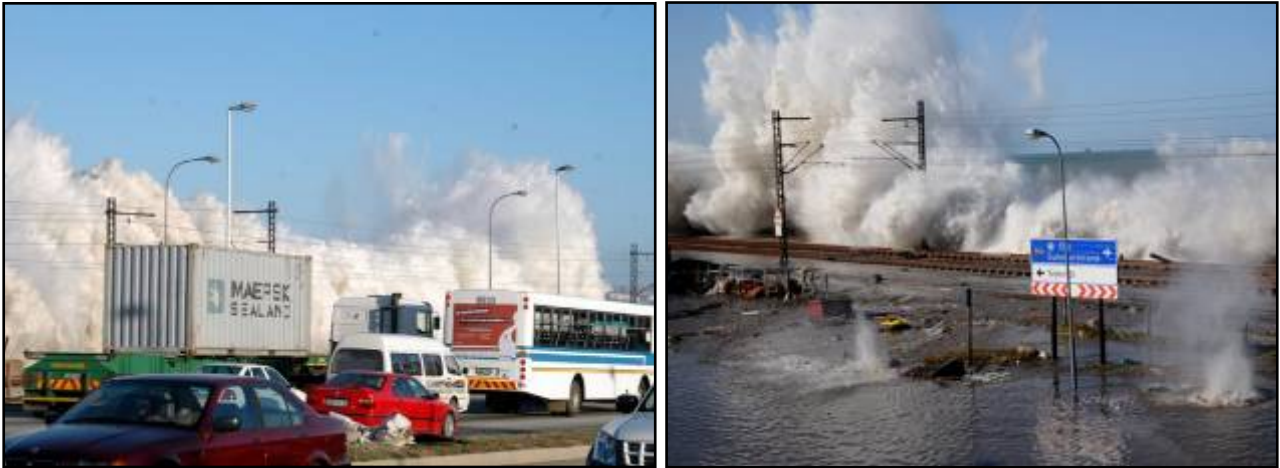
Figure 7 and 8: Severe Wave Overtopping causing Flooding
