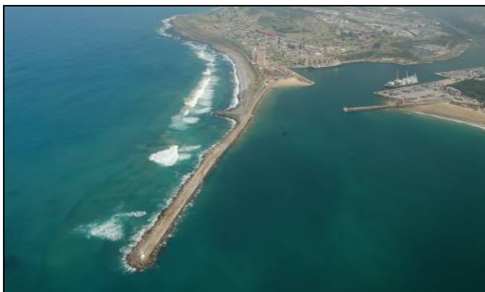
Figure 1: Breakwater Protecting the Entrance of the Port of East London
