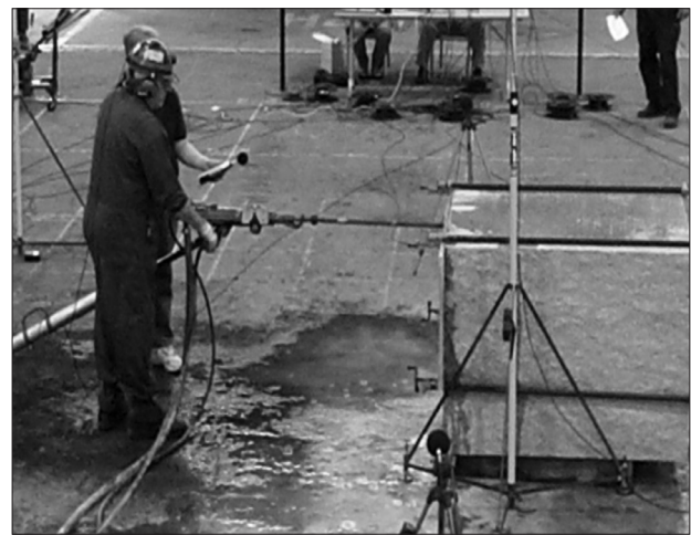
Figure 3—Drilling with the SECO S215
