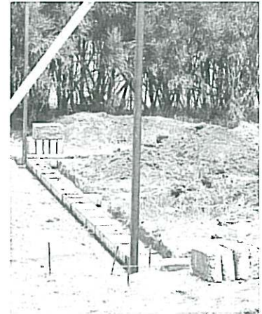
Building foundation walls with stabilised earth blocks
