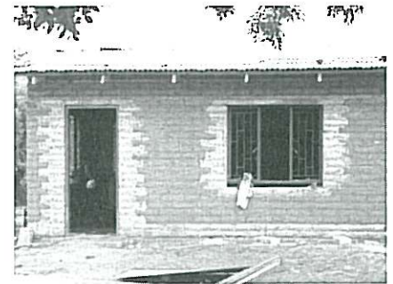
The Lekgophung Development Centre before the walls were plastered
