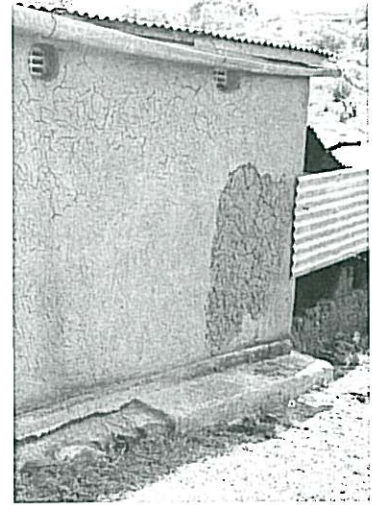
This is an attempt to build foundations after the wall had been built
