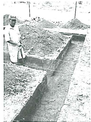
Making trenches for the foundations
