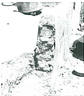
This foundation wall was made from unstabilised earth blocks which have started to collapse
