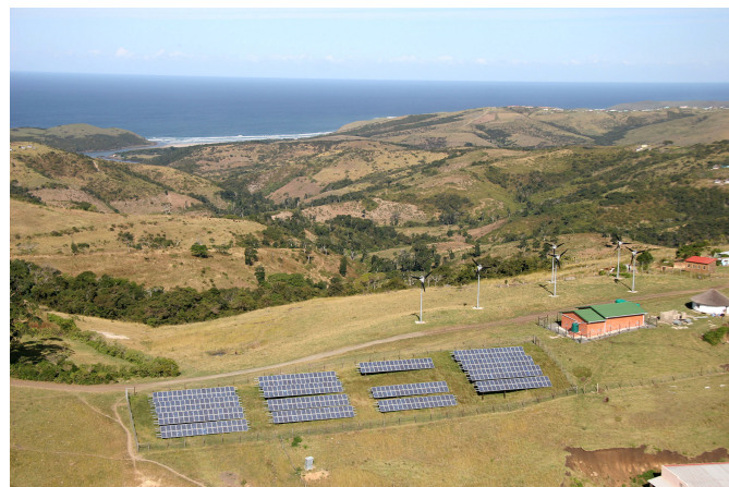
Figure 6: Lucingweni 86 kW hybrid mini-grid
