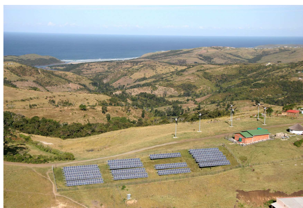
Figure 6: Lucingweni 86 kW hybrid mini-grid
