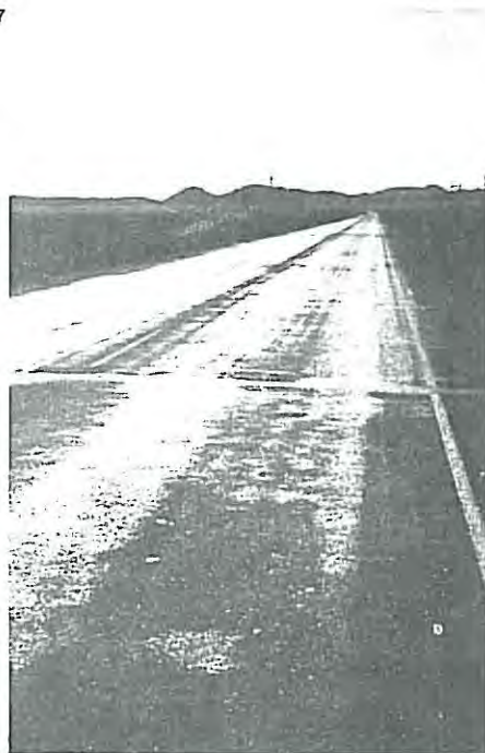
PLATE 19 Cracked and deformed surfacing due to failure of base material.
