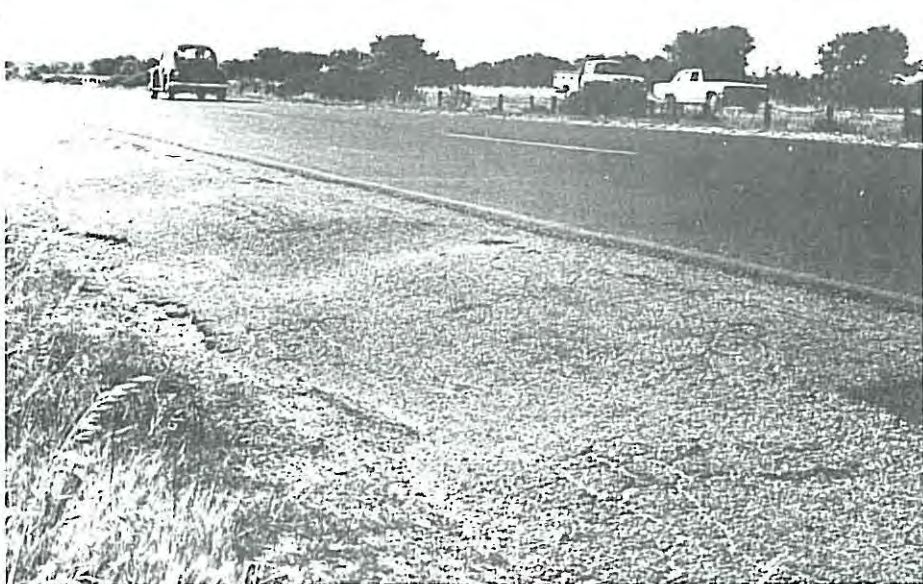
PLATE 10: Borrow 'area' about 150 mm deep near Ariamsvlei, Cape Province, where N is about 40. (Dept. of Transport, Pretoria.)
