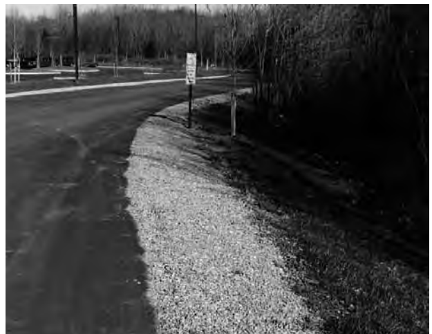
Figure 6.27: Stone aggregate can be placed on the roadside while the shoulder grass establishes itself
