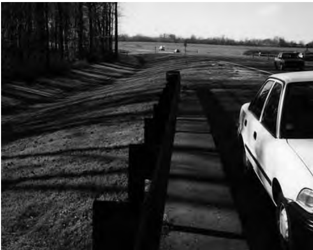
Figure 6.16: Open channel alongside an arterial road
