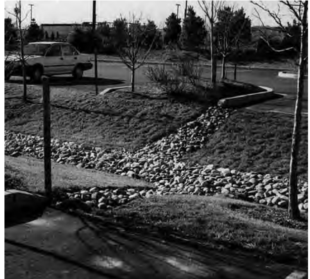
Figure 6.22 (b): Runoff from this parking area is stored in the drainage ways using multiple-outlet drains
