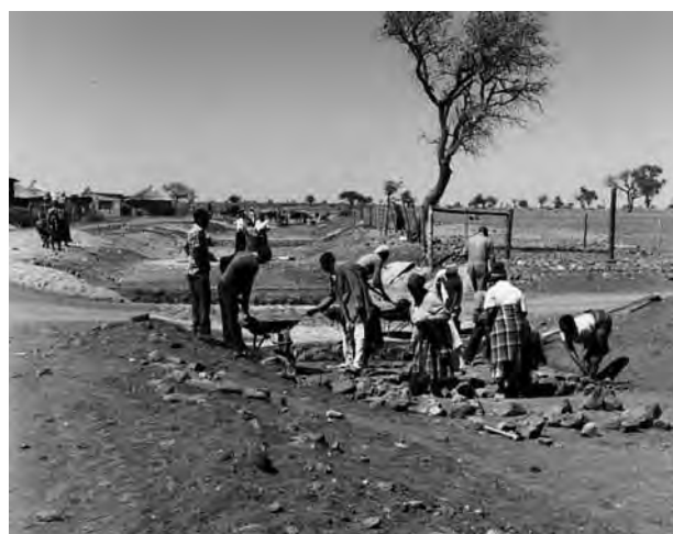
Figure 6.19: Roadside drains of the major system
