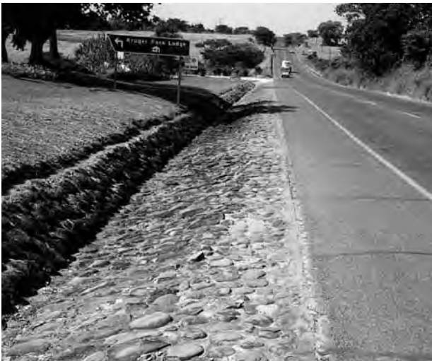
Figure 6.11: A lined open roadside channel
