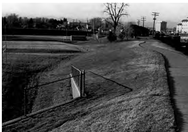
Figure 6.32: These sports fields will act as a detention facility should the watercourse on the right of the picture not be able to convey the flood. Note that the playing surfaces are raised to aid drainage after such an event. The crest of the side weir between the watercourse and the sports fields is designed to accept the excess flow, but is made aesthetically pleasing with a meandering cycle path
