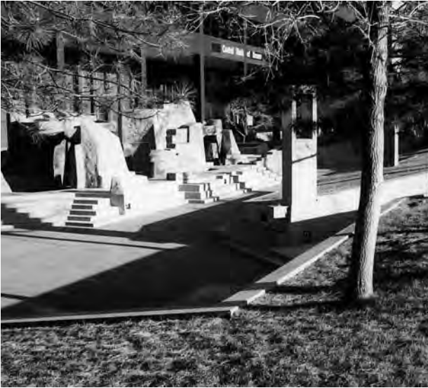
Figure 6.21: This office complex incorporated the entrance to the building in a detention facility. Under normal conditions, this area functions as a pleasant park with water features
