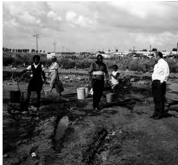
Figure 6.31: This water point has been placed in a low-lying area. Drainage of runoff and water spilled from the point has not been allowed for, and a health hazard has resulted
