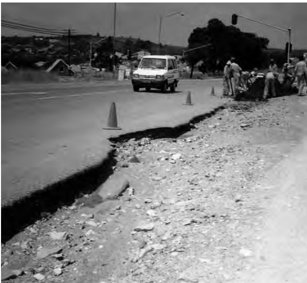
Figure 6.36: Stormwater drainage must occur off the roadway if kerbing is not installed
