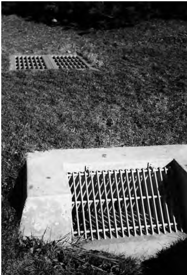
Figure 6.22 (a): Depressed area to store excess runoff
