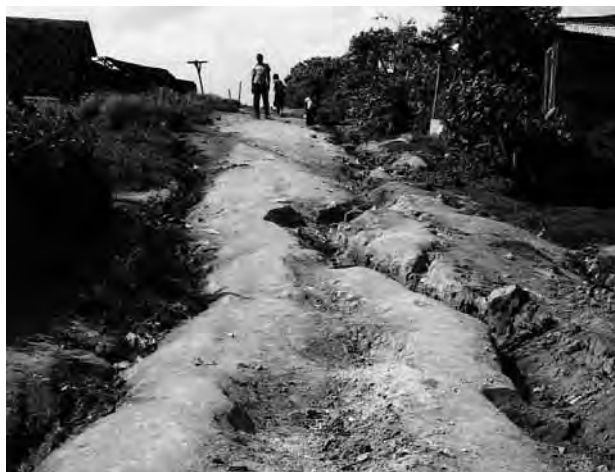
Figure 6.18 (a): Concentration of stormwater drainage in a roadway resulting in major inconvenience to road users
