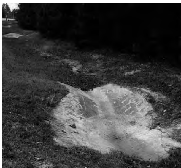
Figure 6.8: Simple drop structures in a residential environment
