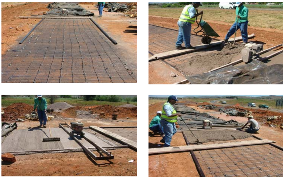
Figure 1: The UTRCP construction process
