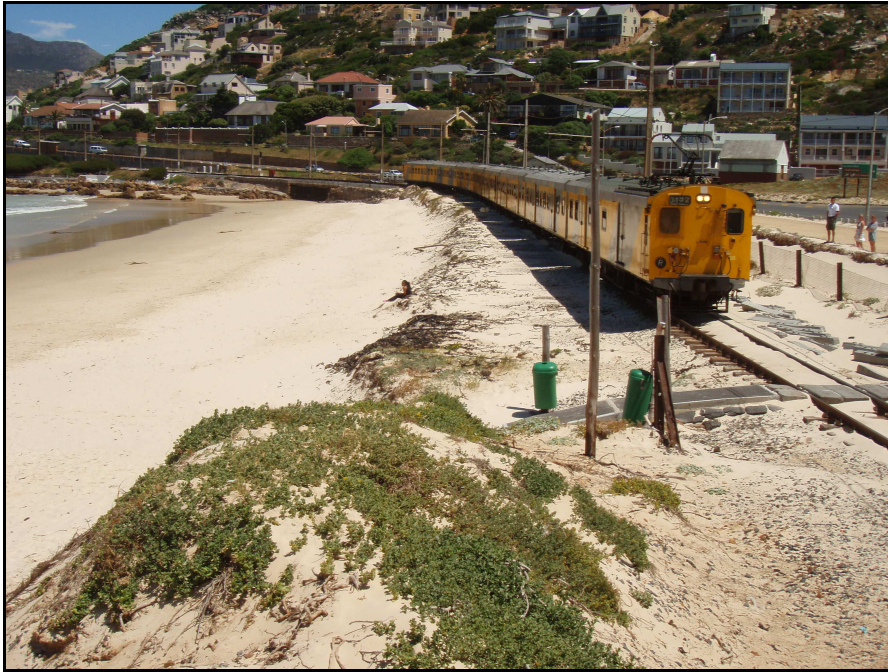
Figure 6: Present SA example of railway line located too close to sea (Photo: A Theron)
