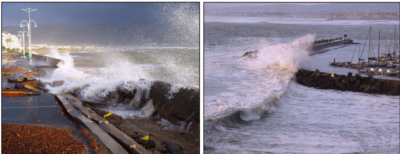
Figure 5: Storm breaching a seawall and overtopping (Cape storm: Sept'08) - examples of existing problems likely to worsen due to climate change (Photos: A Theron)
