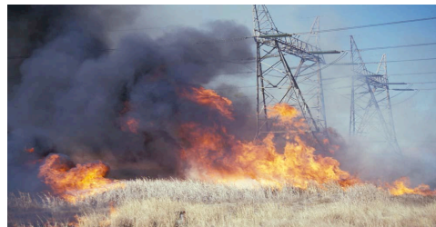
Figure 1. Grassland wildfire near transmission line
