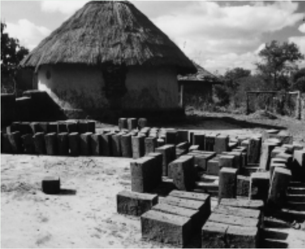
Fig. 15: Traditional house and sun dried earth blocks, Limpopo Province, South Africa.
