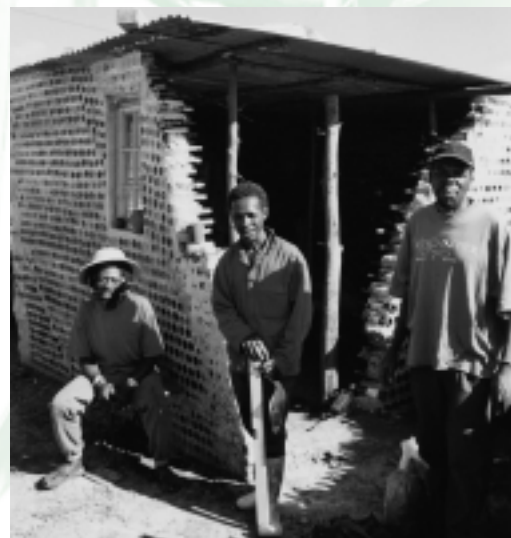
Fig. 13: Informal house built with old bottles, Free State, South Africa.
