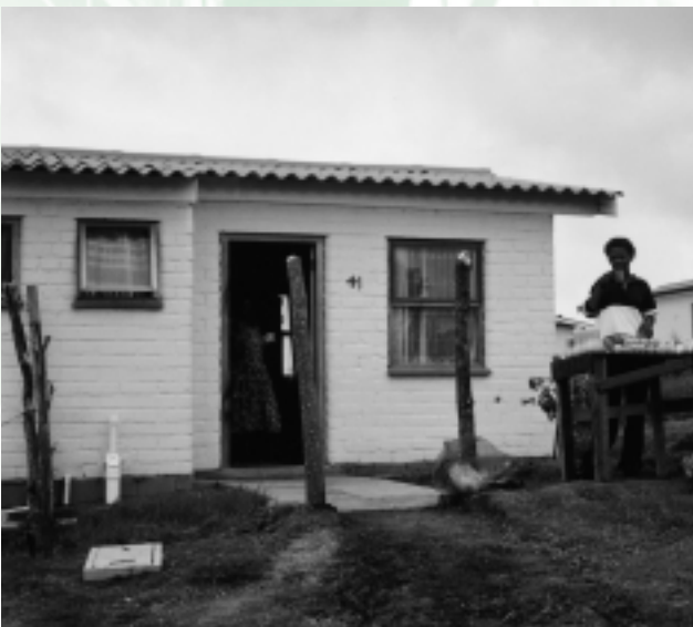
Fig. 16: "Modern" house built with compressed earth blocks, Buffalo City, South Africa.
