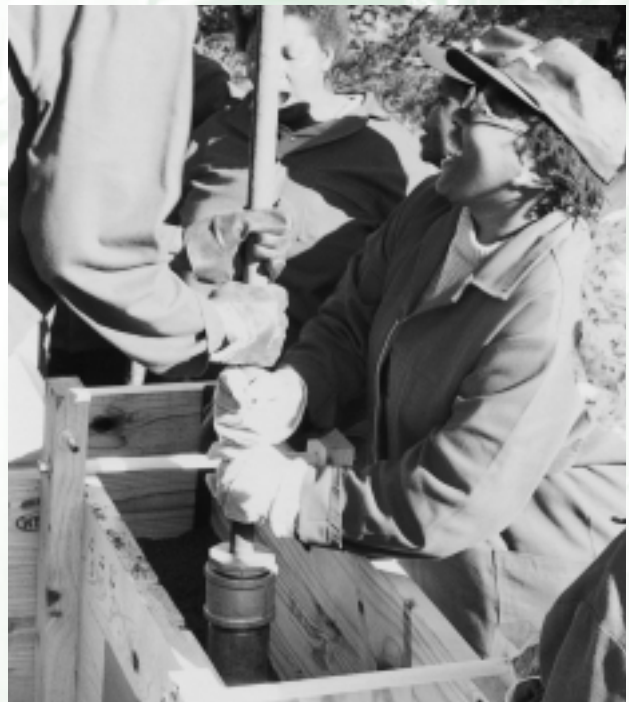
Fig. 10: Women being taught how to build with rammed earth, Johannesburg, South Africa.
