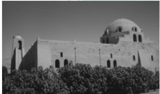
Fig. 14: New Gournah mosque, Luxor, Egypt. Designed by Hassan Fathy and built with sun dried earth blocks.
