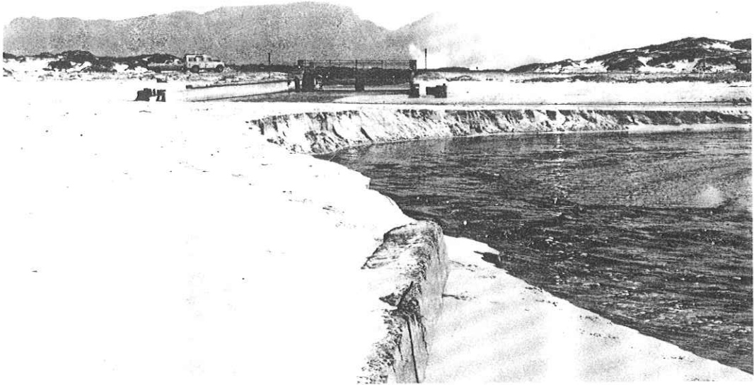
FIG. 4: Mouth of the Zeekoe Canal looking upstream, showing meandering of the channel towards the east. The remains of the eastern concrete berm can be seen in the foreground (ECRU: 80-09-16)
