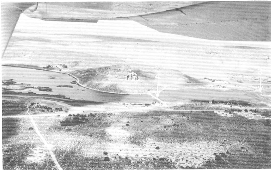
FIG. 22: Narrowing of the Verlorenvlei into a channel, with Obstructions 3 and 4. (Photo: P D Morant, October 1980)
