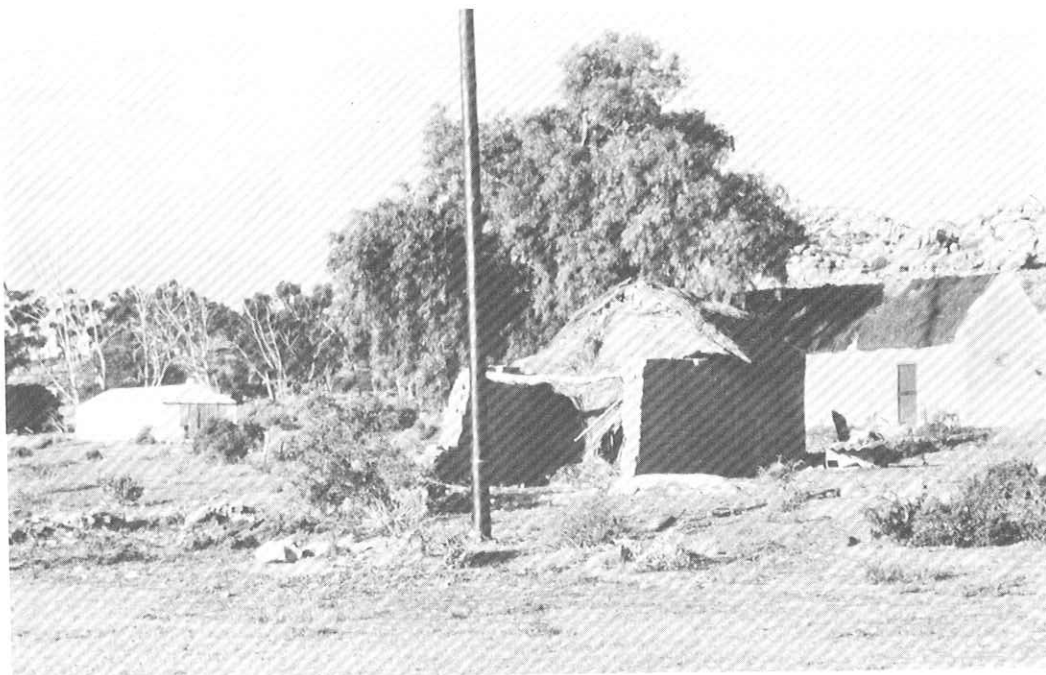
FIG. 3: Powerline support erected in centre of threshing floor. (Photo: S A Sinclair, May 1985).
