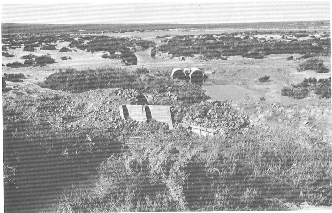
Fig. 10: The seawater supply channel connecting the Papendorp salt pan (in background) with the Olifants Estuary. Note the crude "control gate" consisting of a board and earth dam.
