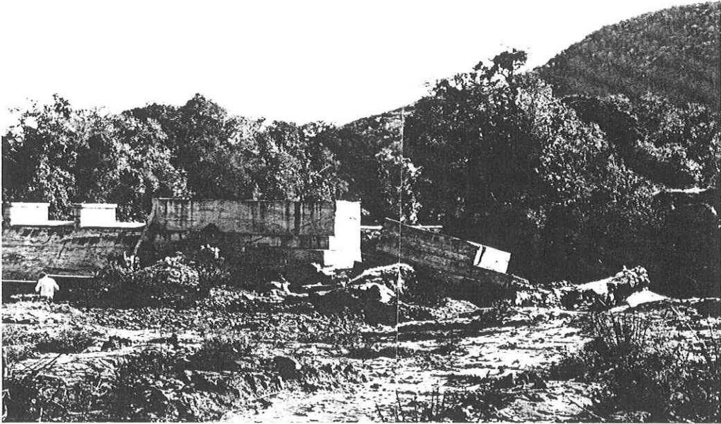
FIG 6: Remains of a weir, damaged in 1979. The weir dammed up the Kowie River for Port Alfred's domestic water supply (ECRU 80-07-06).
