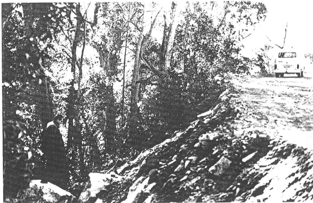
FIG. 8: Encroachment of the embankment of the Onrus to Caledon gravel road onto the Onrus riverbed. Run-off from this road could be a source of sediment to the lagoon during storm conditions. (ECRU, 83-05-19).
