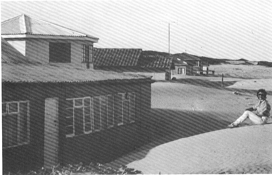
FIG. 21: Sand encroachment and vortex erosion around beachfront houses of Lappiesbaai (1988).
