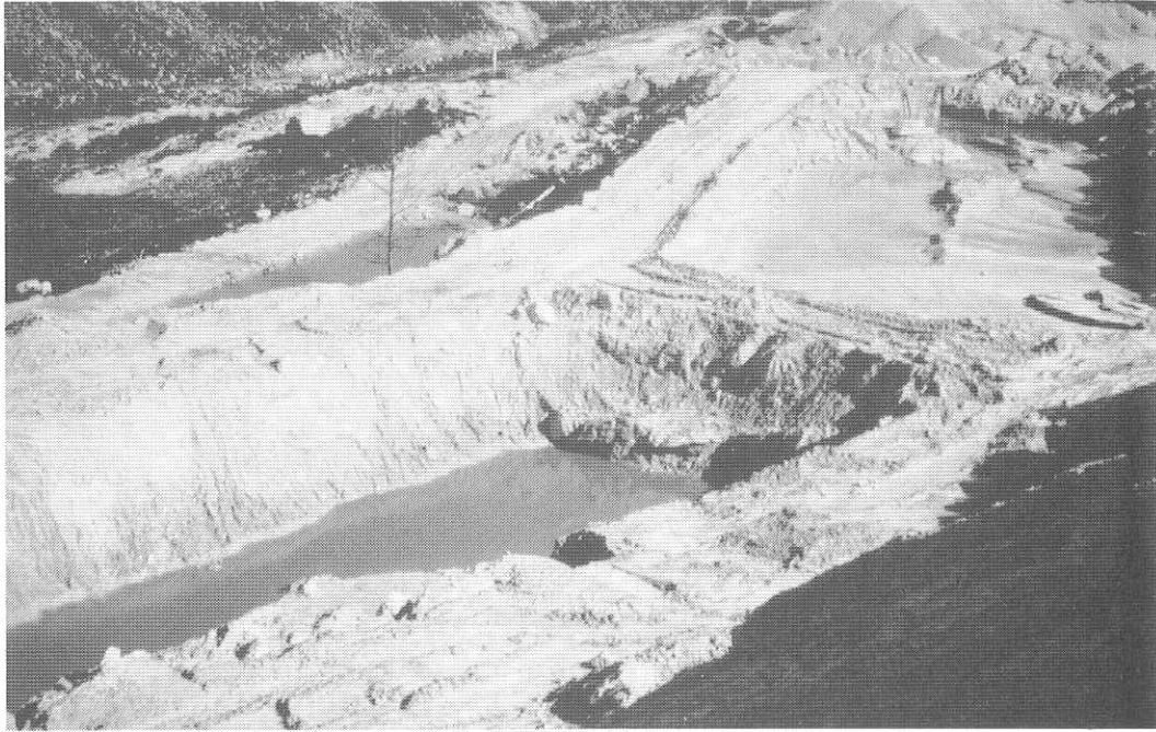
FIG. 13 : Silt traps at the Kogelberg Dam construction site. (Photo: ECRU, 86-09-04).
