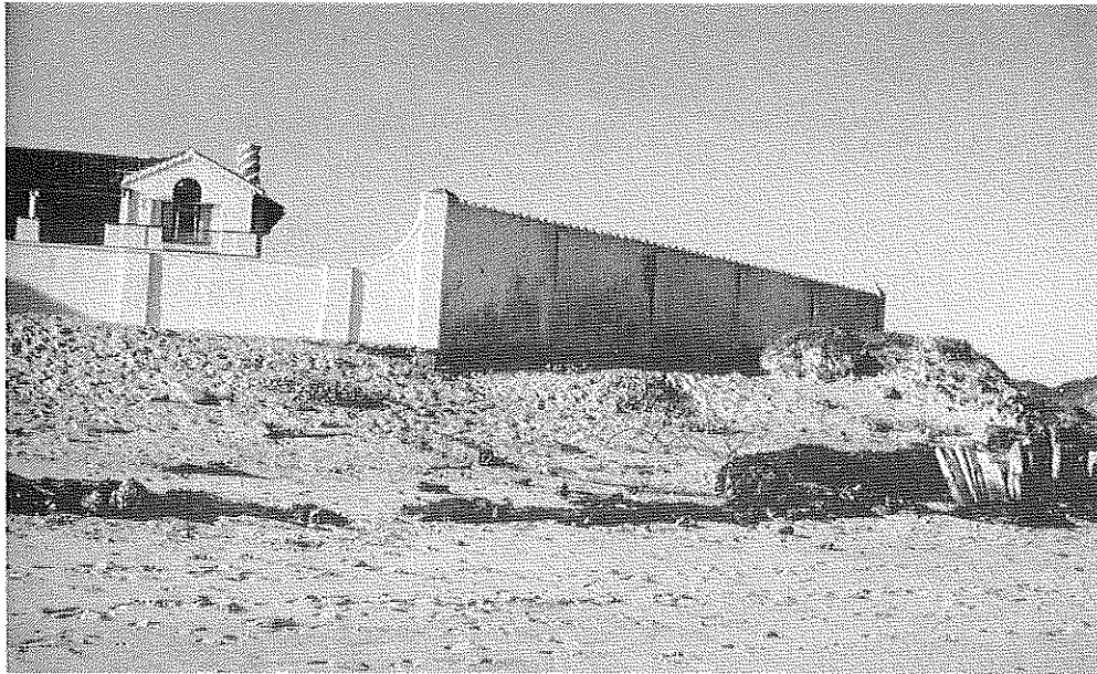
FIG. 12: The historic Zonnekus House on the sandy Woodbridge Island peninsula 400 m north of the mouth of the Diep River Rietvlei system before the great storm of May 1984. (Photo: J R Grindley).
