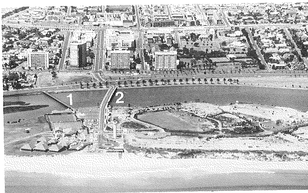
FIG. 20: Aerial view of the two bridges linking Milnerton with the Woodbridge Island peninsula. The Wooden Bridge (1) lies upstream of the new concrete bridge (2). Note Milnerton Lighthouse and Golf Club in foreground. (Photo: ECRU, 87-11-01).
