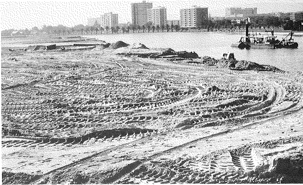
FIG. 10: The lower reaches of Milnerton Lagoon were extensively dredged during 1985 by the dredges visible in the background to provide the sandfill for the Woodbridge Island housing development. (Photo: J R Grindley).
