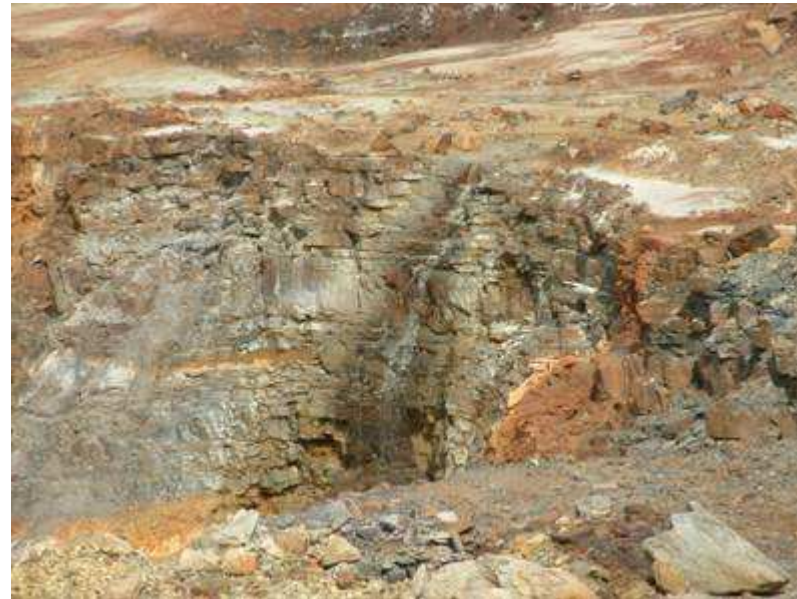
Possible ground water contamination
