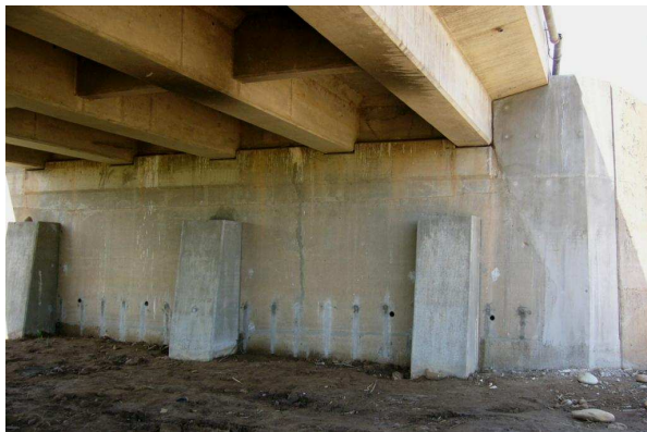
c) Repairs to bridge abutment
