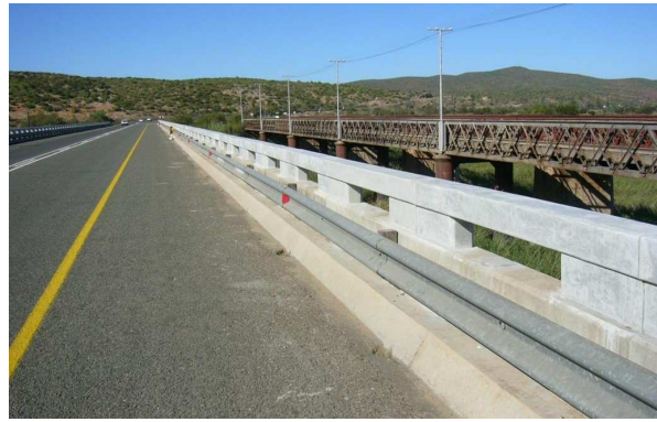
b) Replaced bridge handrails
