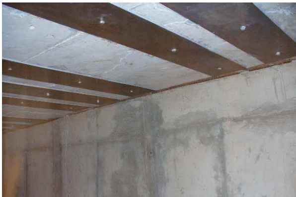
d) Repairs to culvert deck soffit
