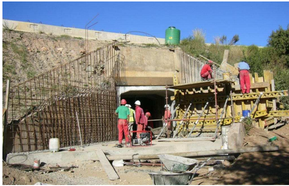
a) Structural repairs to culvert
