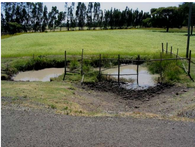
Fig. 6. Ponding of water adjacent to road
