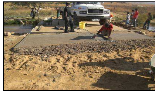
Figure 6: Works in Progress: Esemnteni
