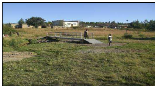
Figure 5: Footbridge in Nordeen – After Intervention
