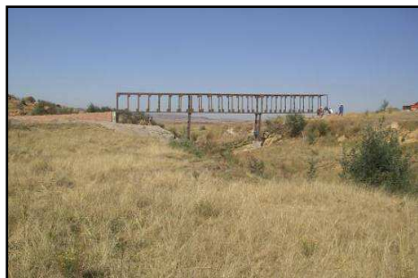
Figure 2: Suncity Mayflower Crossing: Works in Progress
