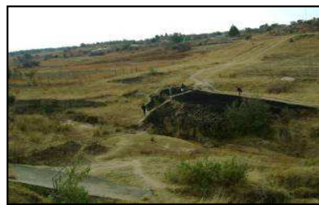
Figure 1: Suncity-Mayflower Crossing-before intervention
