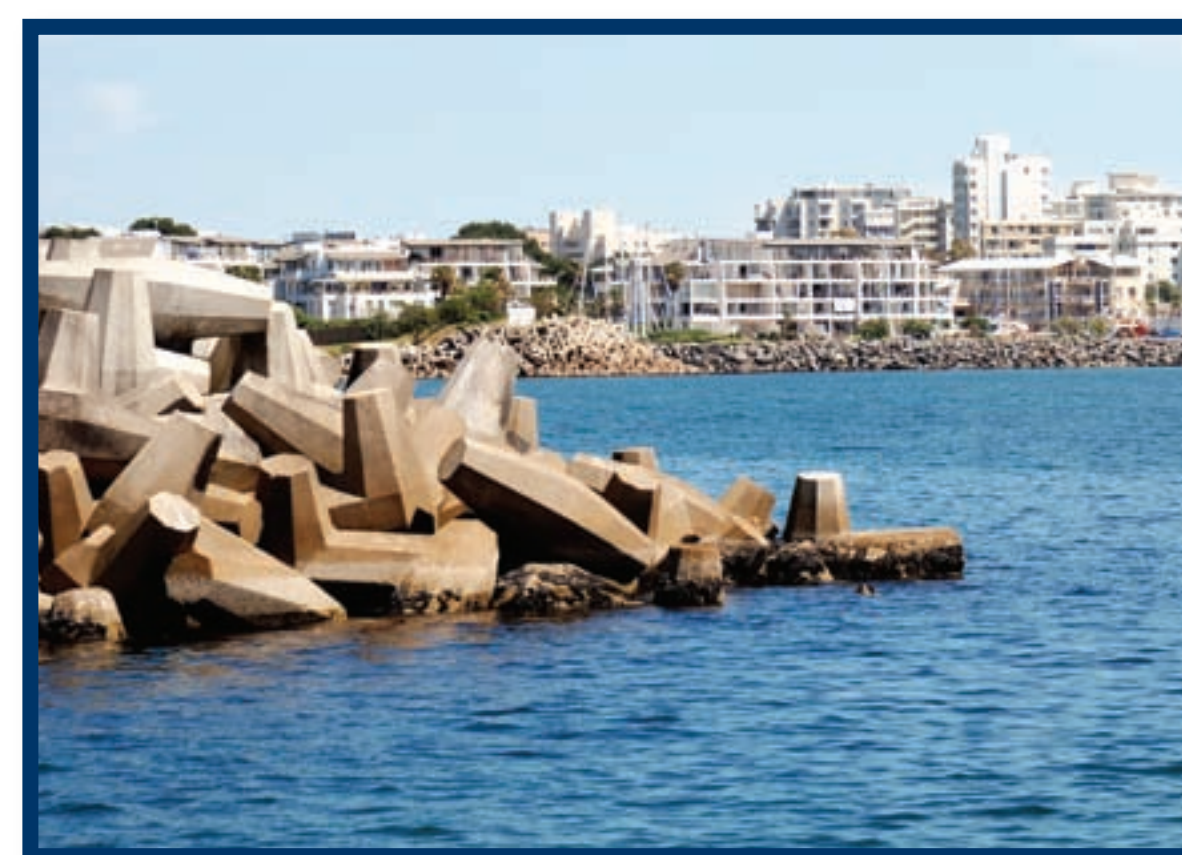
Figure 1: Dolosse protecting Cape Town's harbour. The dolos is a common type of armour unit, invented in East London in the 1960s. The word dolos derives from the Dutch words dollen (playing wildly) and os (ox). While the sea is playing wildly with the dolos through its waves, the numerical project team is 'playing' with them using the game engine PhysXTM. The dolos is made from unreinforced concrete and
